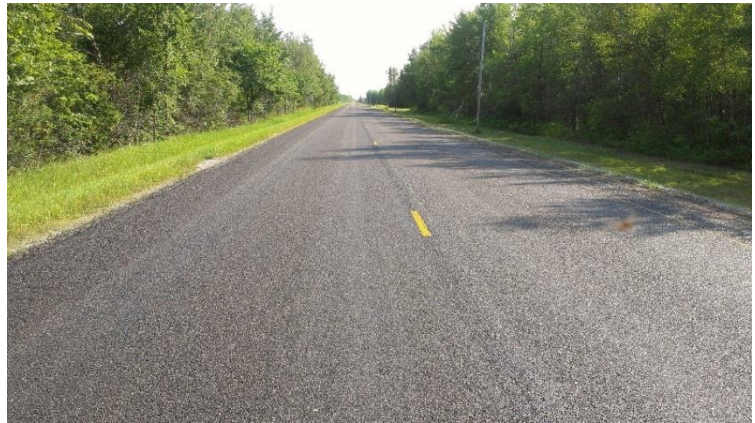
Figure 2 - TH 89 after Placement of Chip Seal
